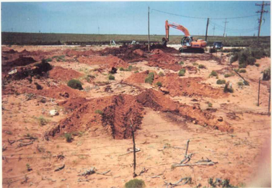
Phase I – Digging Shallow Trenches
