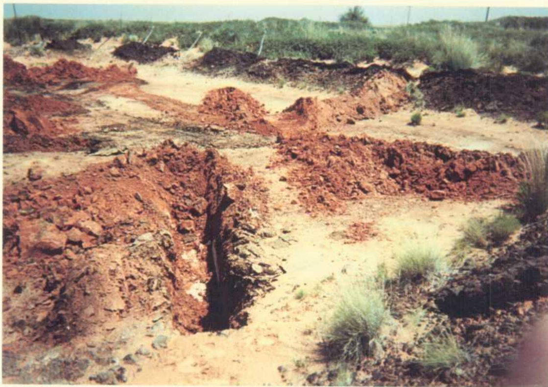
Phase I - Inspection Trench – Showing Non-Affected Soil
