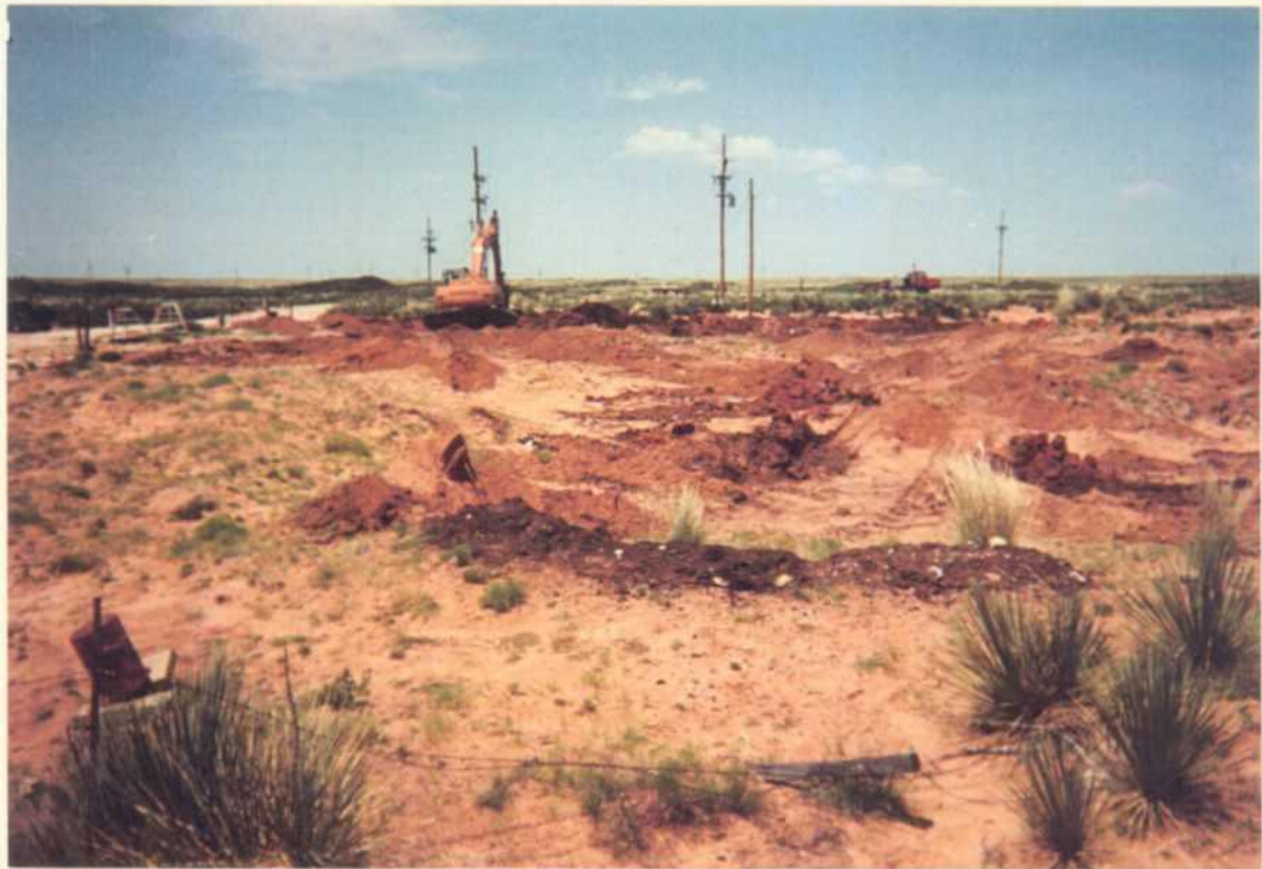
Phase I – Digging Shallow Trenches
