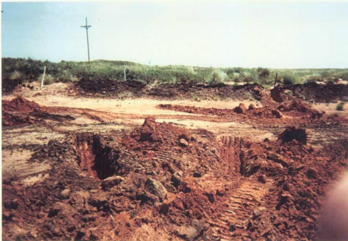
Phase I - Inspection Trench – Showing Non-Affected Soil
