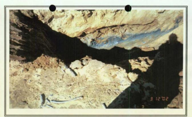
Photo 11. Excavation #9 – Stained soil in side wall with dark staining at depth.
