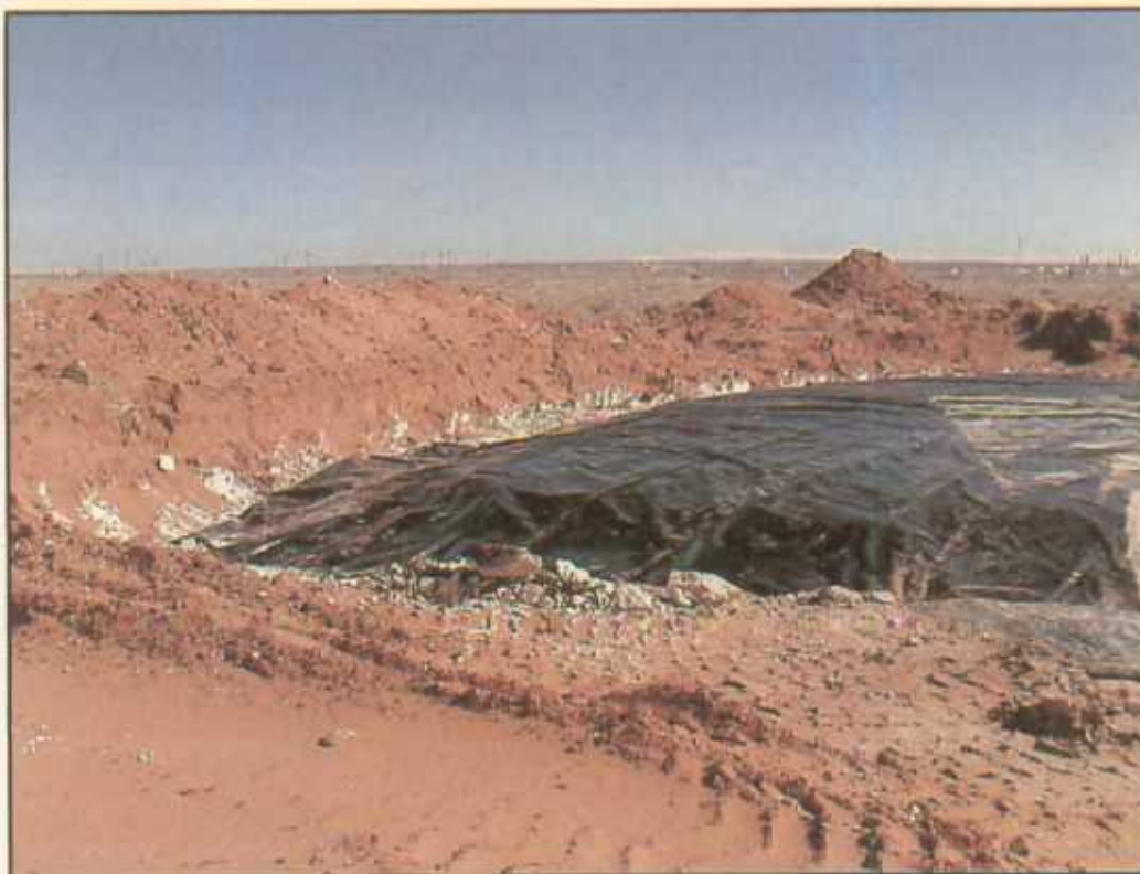
Installed Liner
