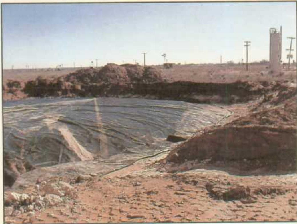
Installed Liner
