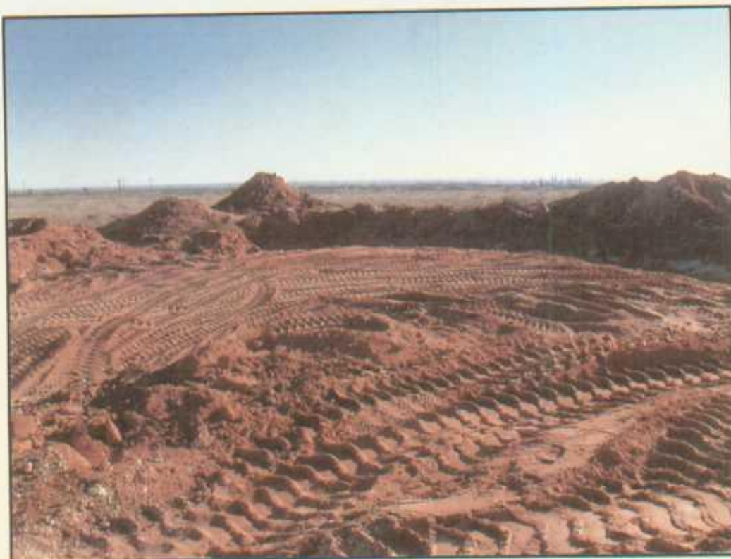
Sand Cushion on Top of Liner
