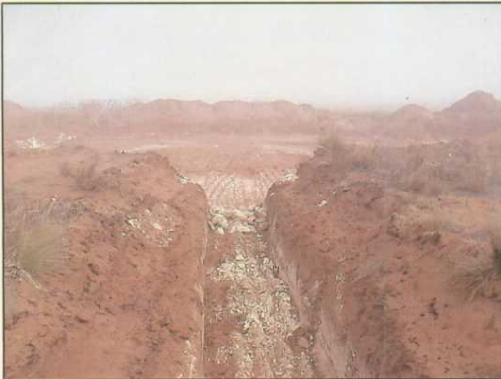
Excavation Prior to Liner Installation
