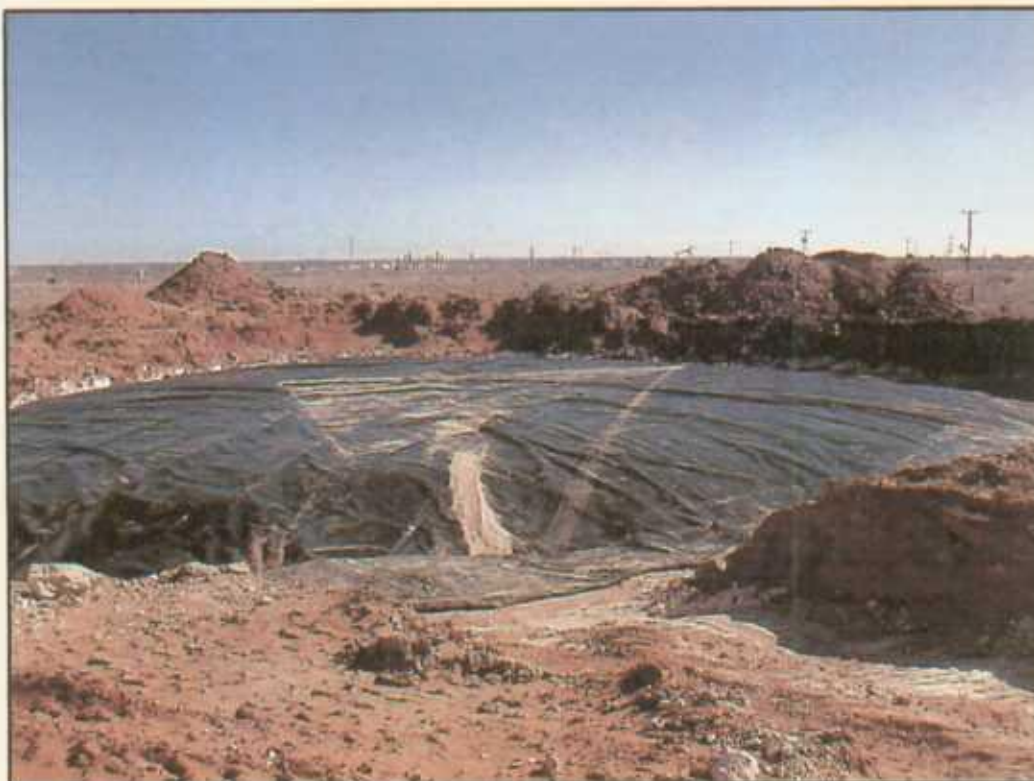
Installed Liner
