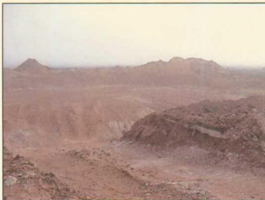
Excavation Prior to Liner Installation
