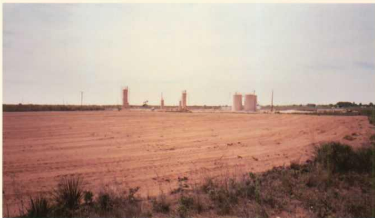
Photo 14. Completion of backfill and site grading (04/29/03).
