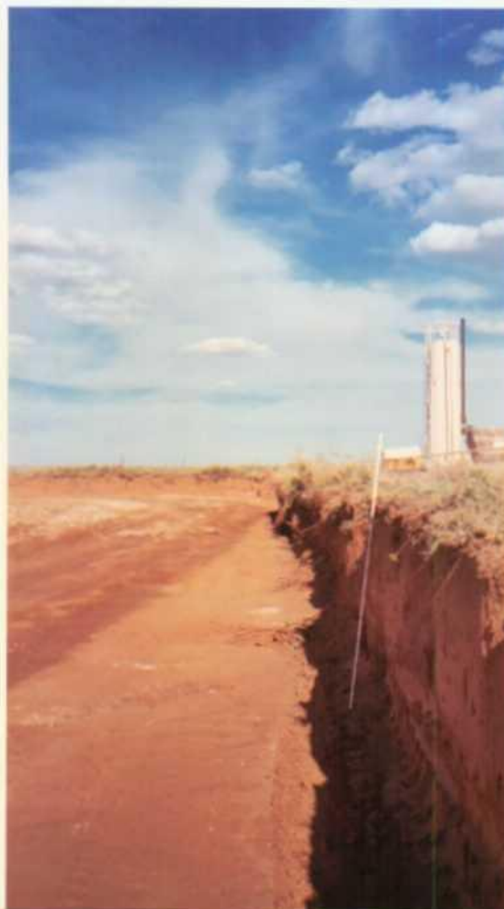
Photo 8. Sub grade elevation for clay layer (note six-foot rule) (04/14/03).
