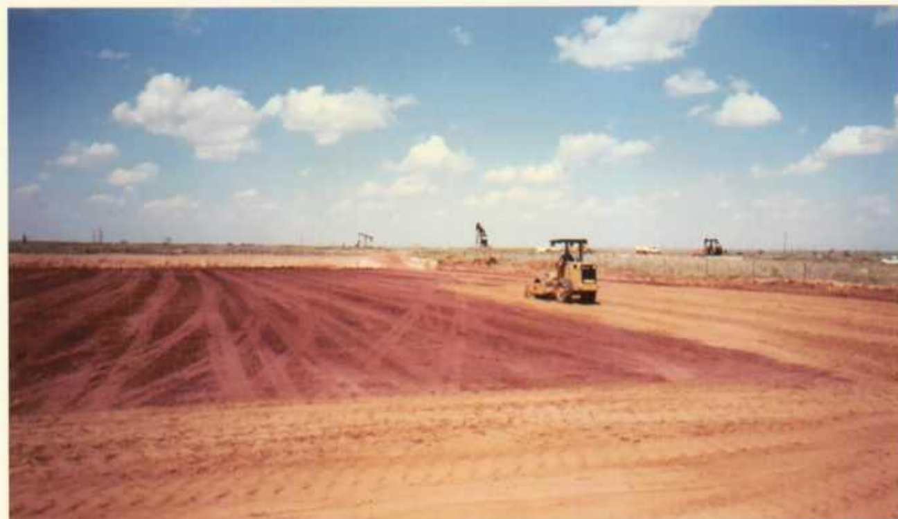
Photo 12. First lift of cover soil over clay layer (04/22/03).
