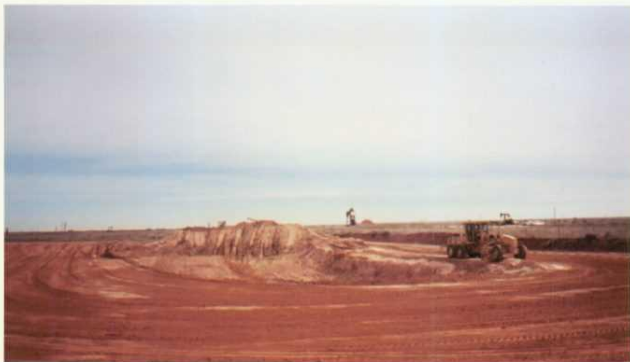
Photo 3. Backfilling of main pit and site grading (04/10/03).
