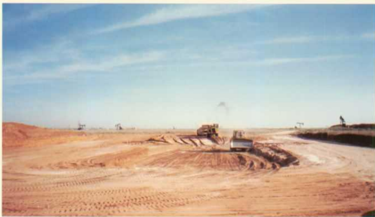
Photo 4. North pile removed; completion of backfill of main pit (04/11/03).
