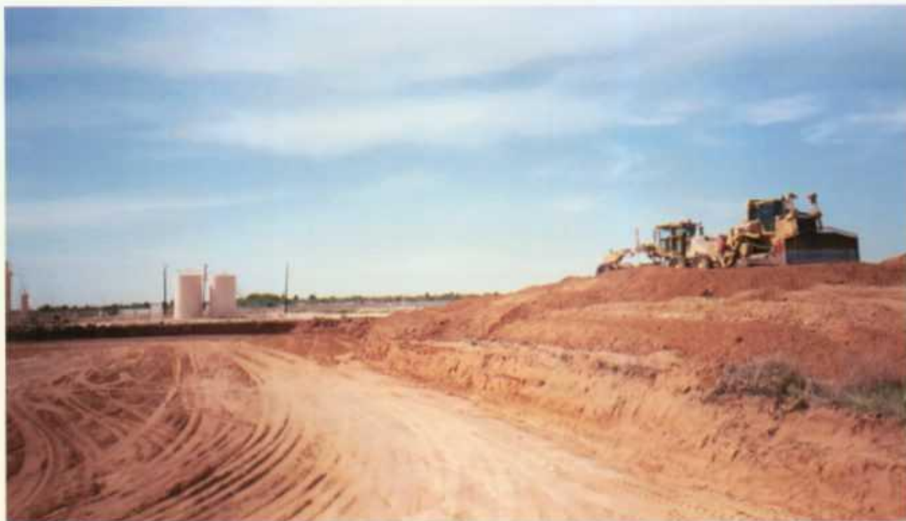
Photo 5. Site grading and stockpiling of cover soils (04/11/03).
