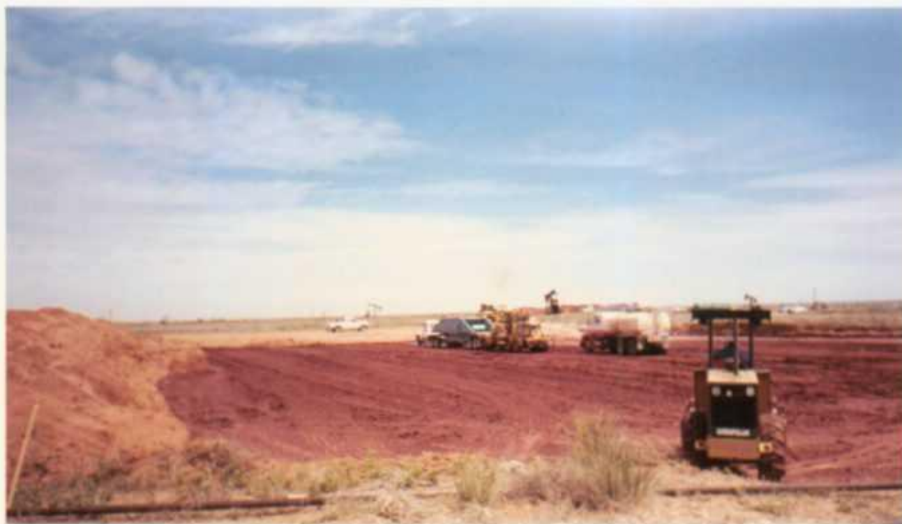
Photo 9. Construction of clay cover (04/18/03).
