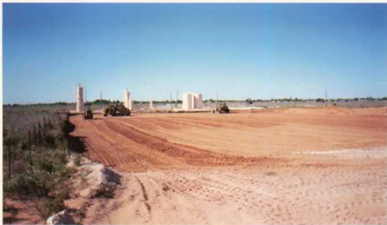
Photo 13. Placement of compaction of cover soils (04/24/03).
