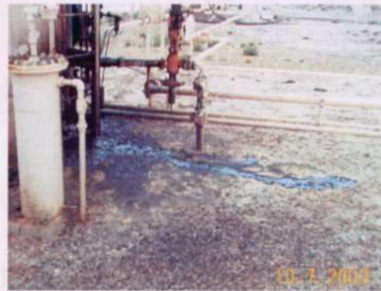
#4 Penroc State 11-23 battery #1-Oil and water observed being discharged to ground surface.
