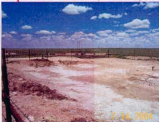
Penroc Harris State #5- Looking East-Southeast- picture shows salt staining.
