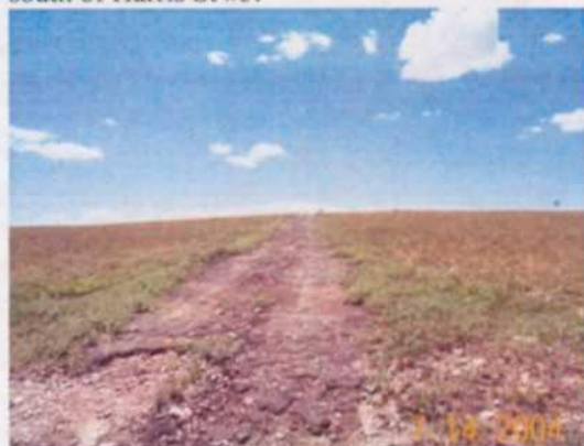
Road leading out of Harris #5. Picture shows where oil and tank bottoms were placed on road.
