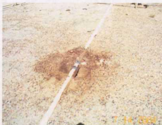
Penroc Battery State 11-23 picture shows gas line. Line was noted to be leaking and a slight H 2 S smell was noted. Did not sample for safety reasons. Battery did not have H 2 S signs.
