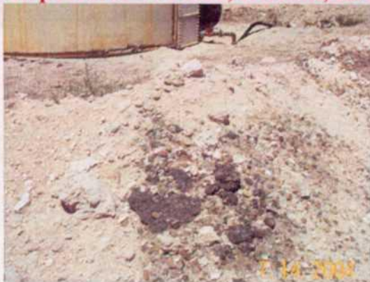
Penroc Battery State 11-23 berm. New dirt has been placed over old berm. Picture shows old oily dirt.
