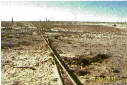
Picture # 1489- Flow line leak site 300 feet west of Lovington City water well #18. Picture looking west. At time of visit soil had a distinct hydrocarbon odor and exhibited gross staining. Most of the spill area was covered with sand.
