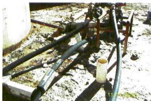
Picture # 1436- North side of pumps looking south. Soil is wet and gross salt water staining observed.
