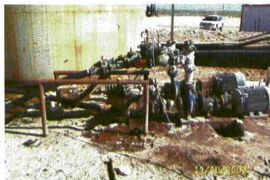
Picture # 1435- Saga SWD tanks and centrifugal pumps inside of berm. Picture taken from west side looking SE. At time of site visit these pumps were leaking water onto the ground surface.
