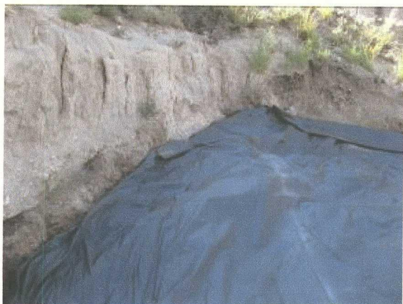
Photo #11 A corner of the PVC liner in the floor of the excavation.
