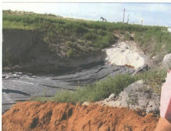
Photo #8 View to the southeast of the PVC liner on the floor of the excavation.
