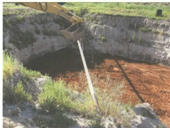
Photo #6 View of sand being backfilled into the floor of the excavation.
