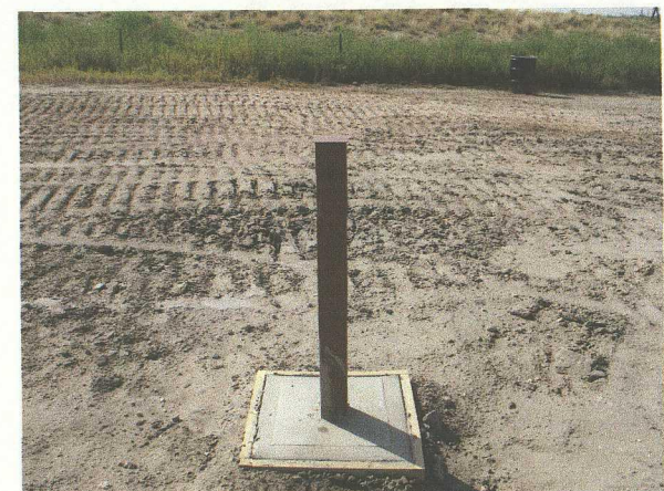
Photo #24 Monitor well TMW-1 completed with steel riser and concrete pad.
