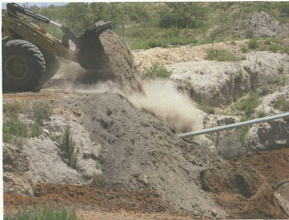
Photo #19 Begin backfilling the stockpiled material at the site.
