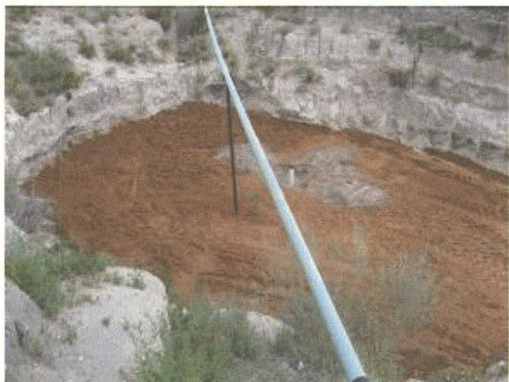
Photo #5 The excavation floor, monitor well TMW-1 has been shortened in order to install the PVC liner.
