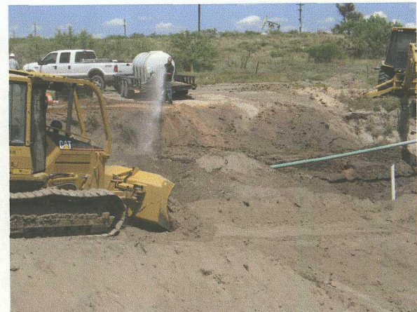
Photo #22 Hosing down the stockpiled material as it is being backfilled into the excavation.
