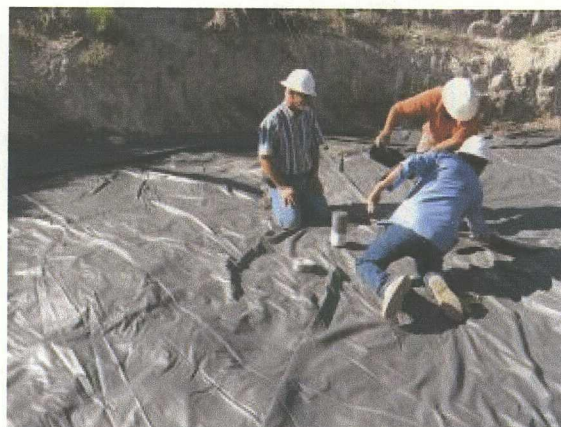
Photo #10 Laying the PVC liner on the floor of the excavation around monitor well TMW-1.
