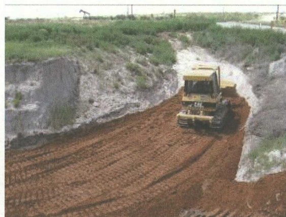
Photo #4 View to the southeast of sand being backfilled into the excavation.
