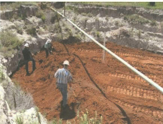
Photo #17 View to the east of sand being placed below the pipeline.
