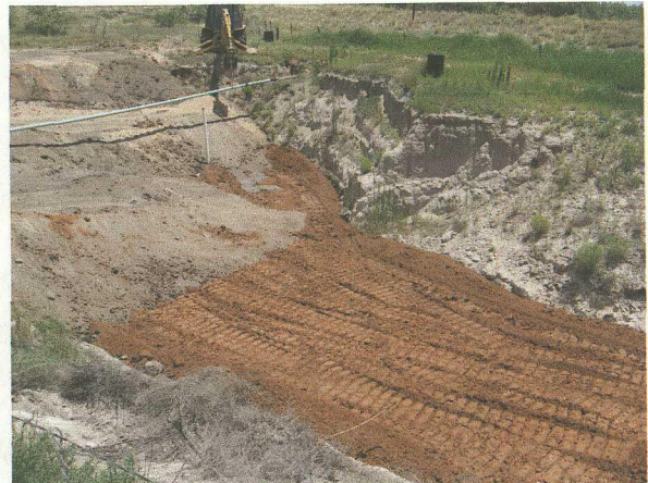
Photo #20 View to the northeast of stockpiled materials being placed over the sand at the excavation.
