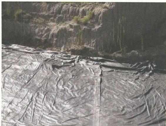
Photo #9 Central portion of the excavation with the PVC liner on the excavation floor.
