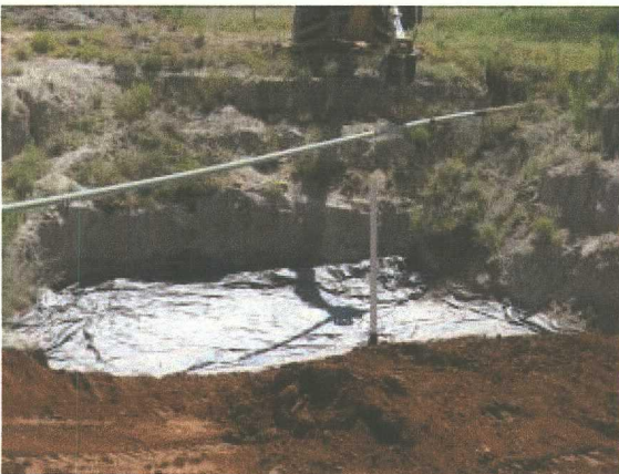
Photo #15 Placing sand on top of the liner. Monitor well TMW-1 is visible in the center of the photograph.
