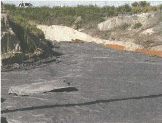
Photo #13 View to the southeast of the PVC liner at the floor of the excavation.
