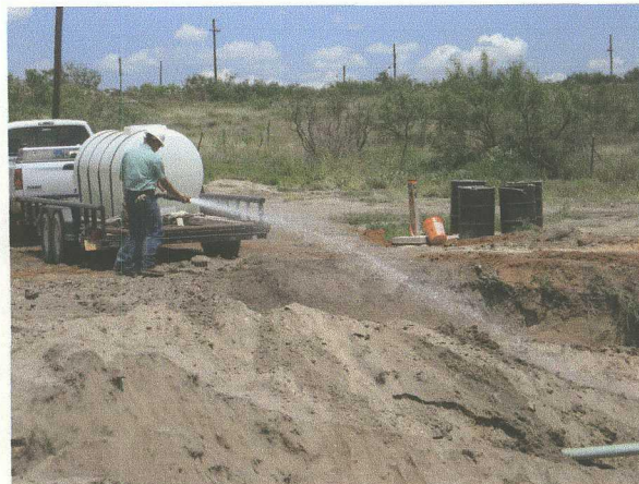
Photo #21 View to the northeast; hosing down the stockpiled material as it is being backfilled into the excavation.
