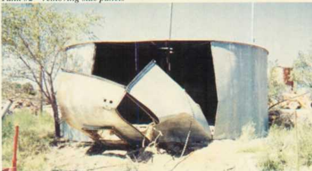
Tank #2 – removing side panels
