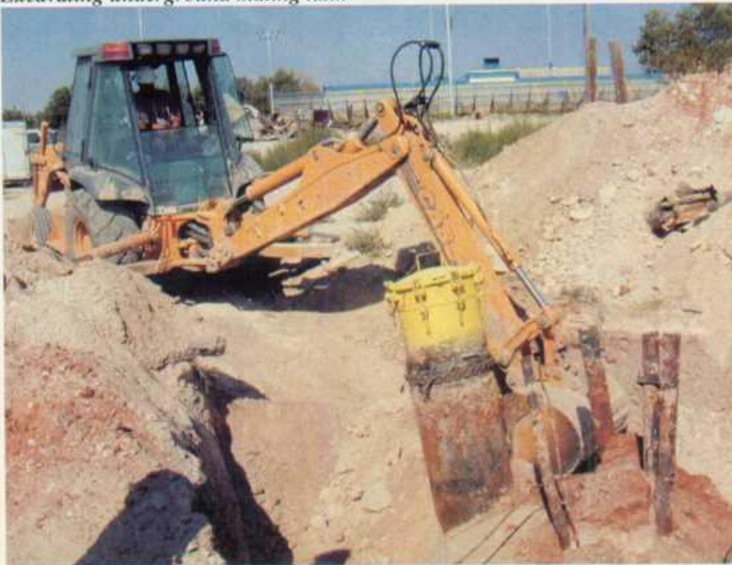
Excavating underground mixing tank
