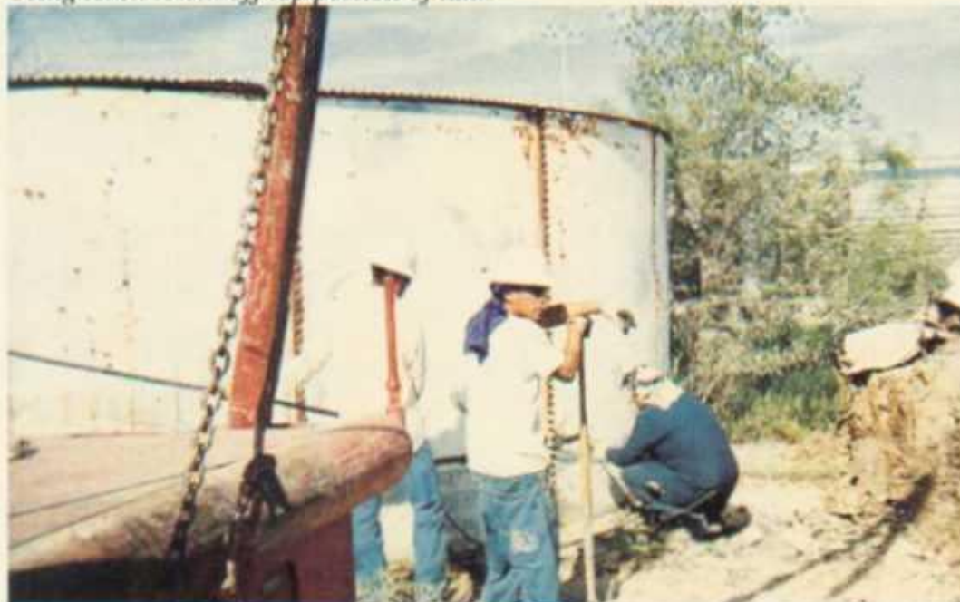
Using torch to cut off top portion of tank
