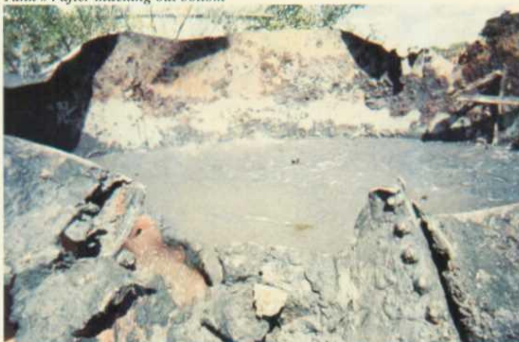
Tank #4 after mucking out bottom
