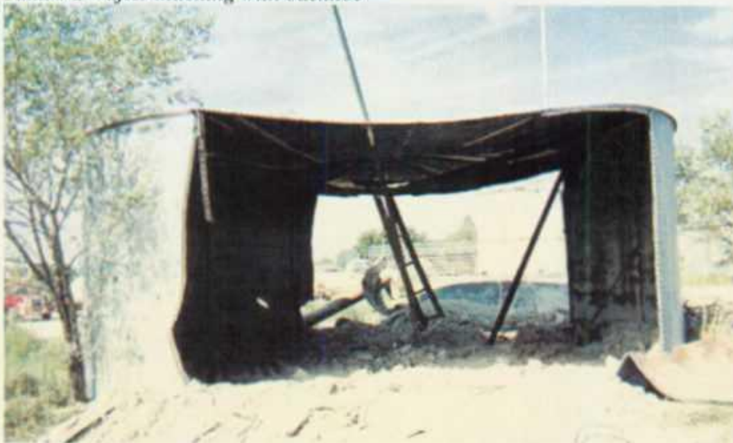
Tank # 2 – after mucking with backhoe
