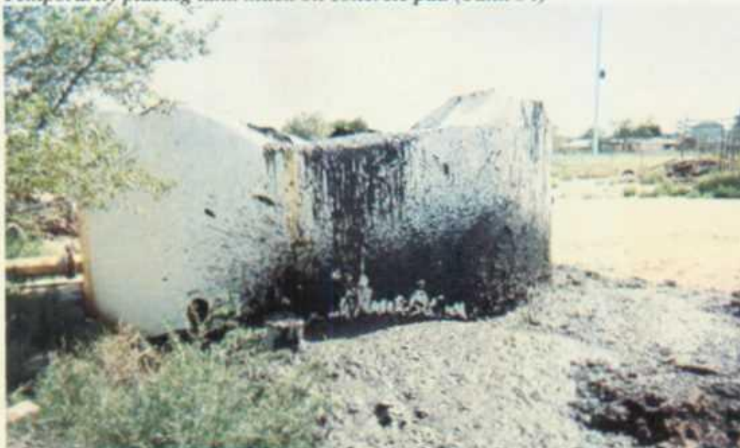
Temporarily placing tank muck on concrete pad (Tank #4)
