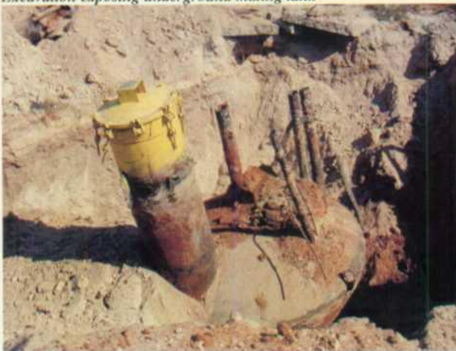
Excavation exposing underground mixing tank
