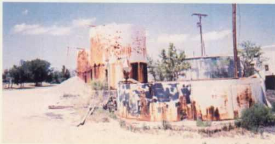
Picture 9. A corroded 250-barrel blender tank (bolted)
