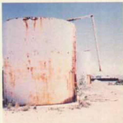
Picture 4. A 500-barrel welded tank
