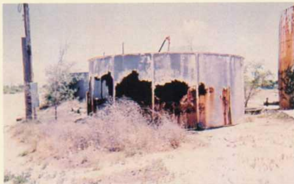
Picture 6. A highly corroded 250-barrel bolted tank
