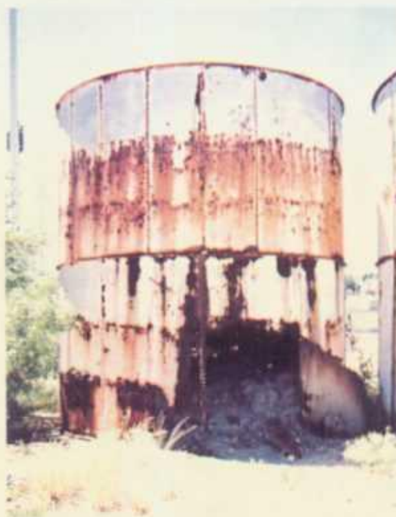
Picture 5. A highly corroded 500-barrel bolted tank
