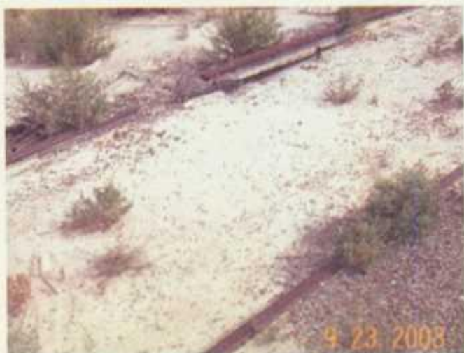
Photo 13: Railroad siding is corroded. Surface drainage from Runco drains across this location
