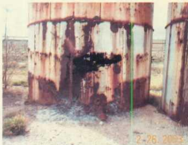
Photo 20: Mud tank along drainage that is corroded.
