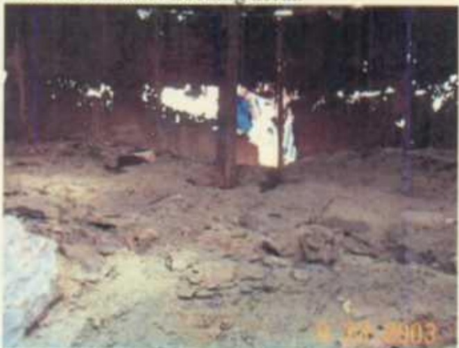
Photo 3: Mud tanks are rusted and corroded.
