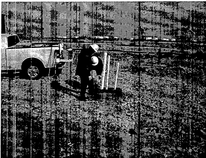
Figure 3: Bentonite being placed around Lysimeter 1 casing and associated Tensiometer casings. MW-1 is visible to the upper right of Lysimeter 1 casings.
