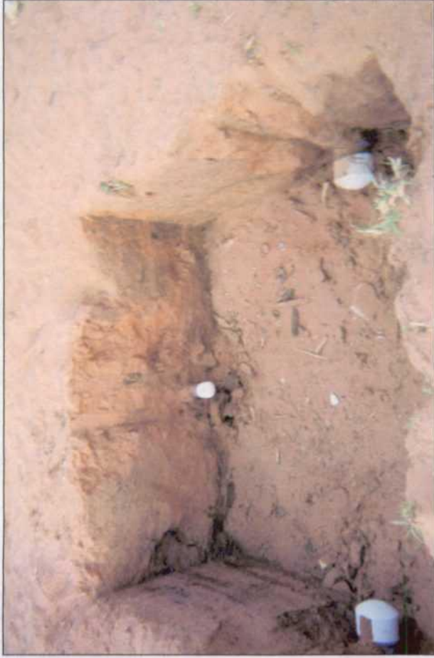
Box and connections removed 11/5/2003
