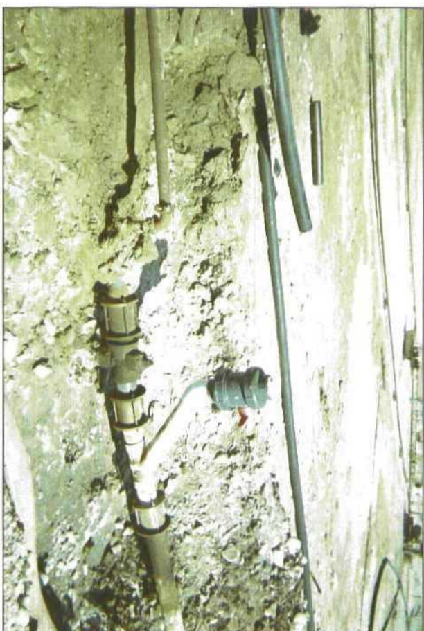
junction box removed; old plumbing
