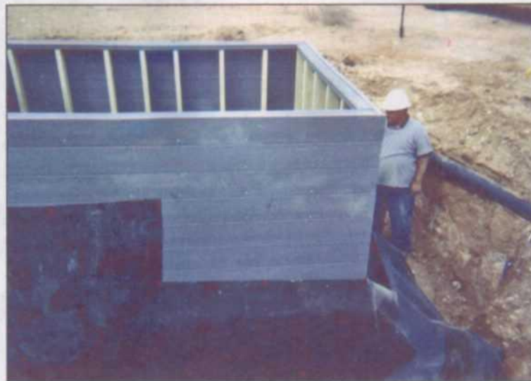
Box Construction With Plastic Liner
