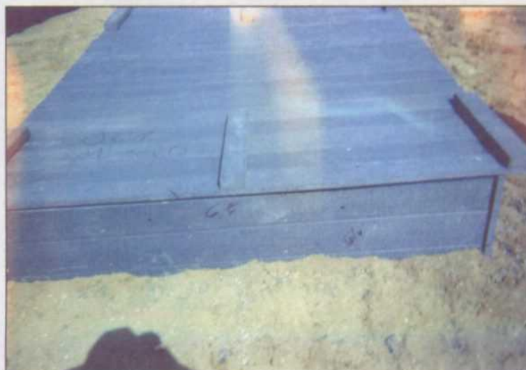
Completed New Junction Box
