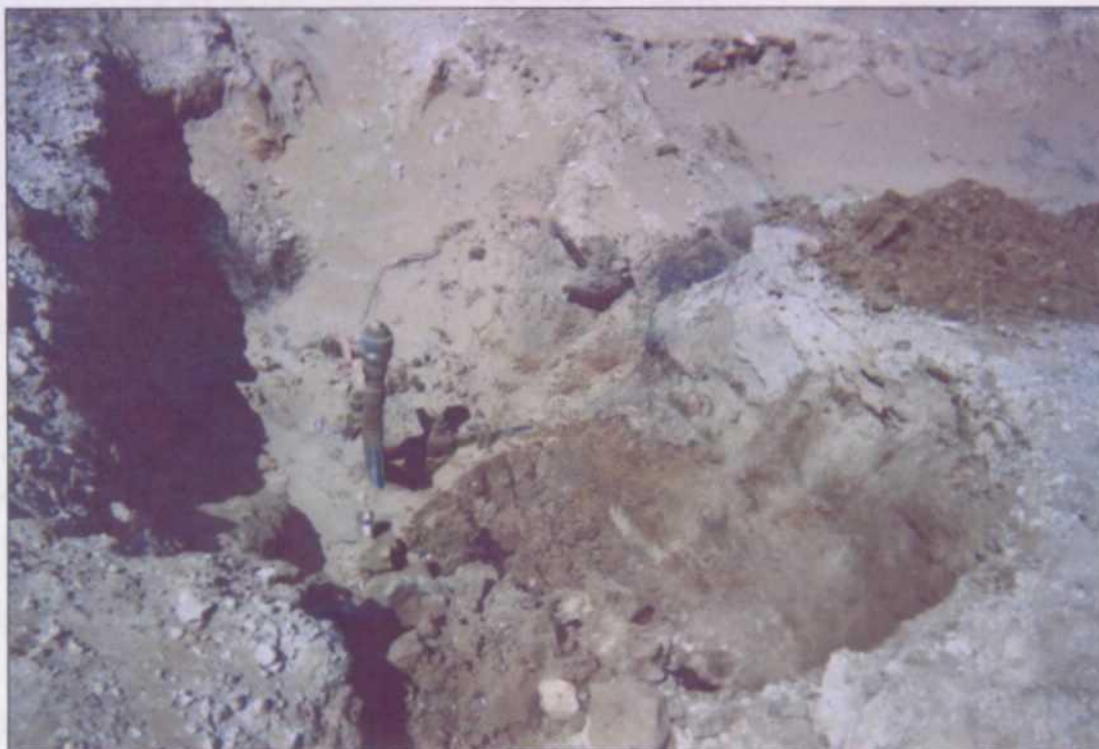
Before Excavation, After NORM Removal
