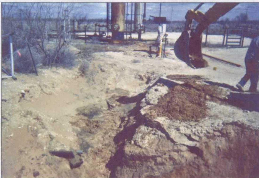
Beginning Impact Excavation
