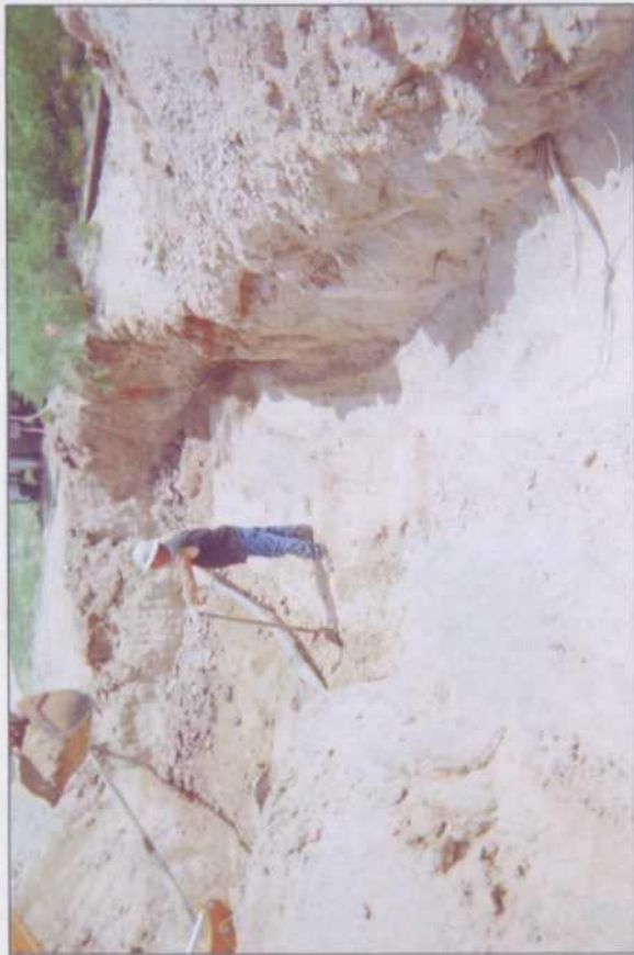
backfilling excavation
