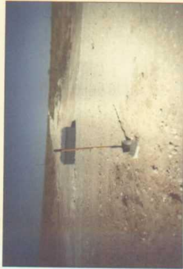
Identification plate marking clay barrier
