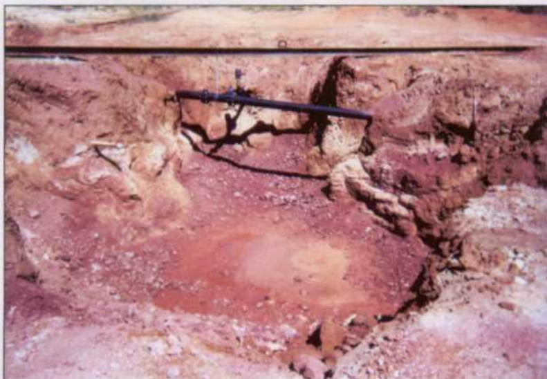
Clay Liner in Excavation
