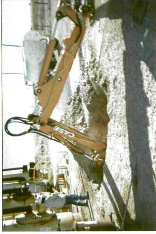
backfilling delineation trench
