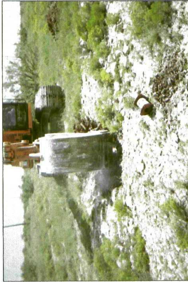
beginning junction box delineation & excavation
