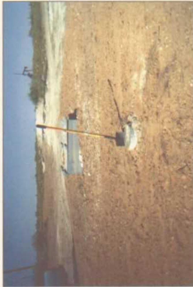
Backfilled with Clay Identification Plate in Foreground; New Box 15 ft North of Old Junction Box
