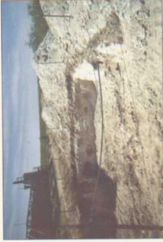
30 x 23 x 12-ft Excavation Before Installing Clay Barrier (August 2003)
