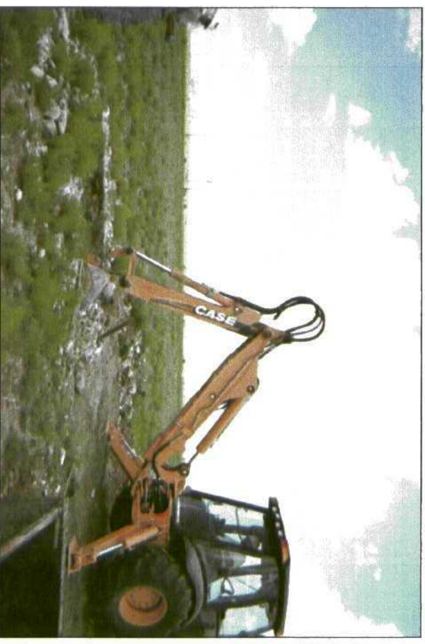
delineation trench at former box site
