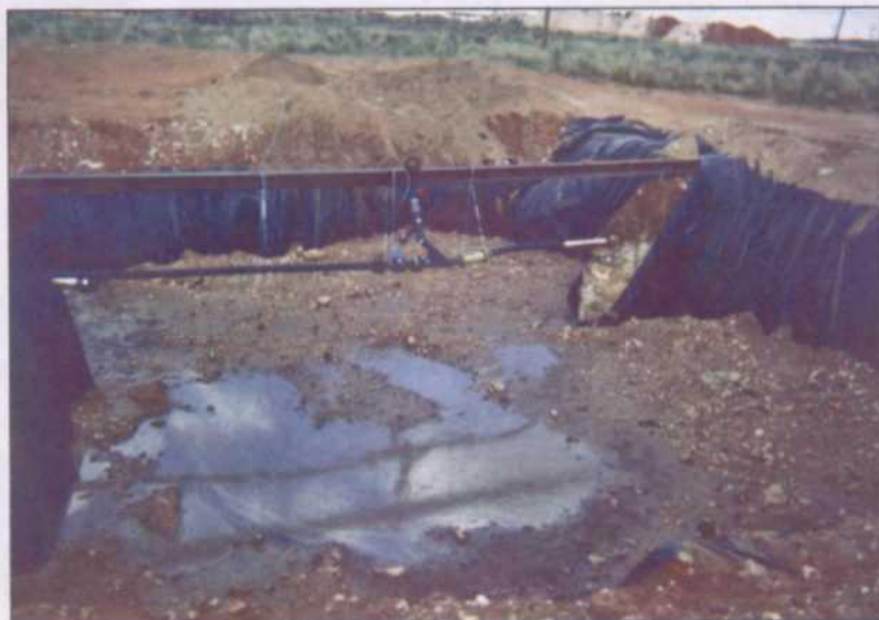
Backfilling & Water-packing Excavation
