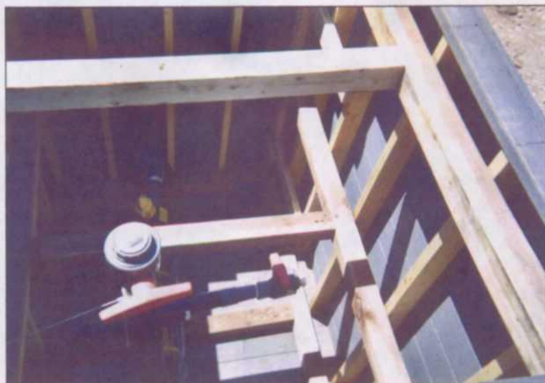
Junction Box Construction
