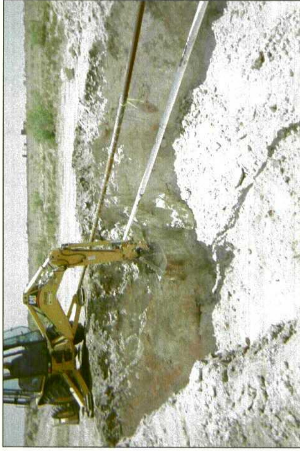
sampling final 30 x 30 x 12 ft excavation
