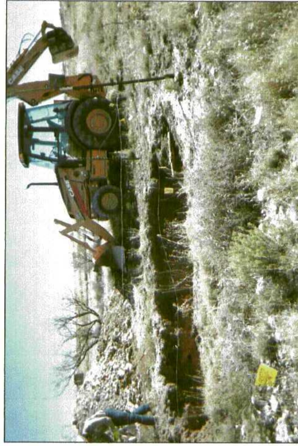
backfilling trench
