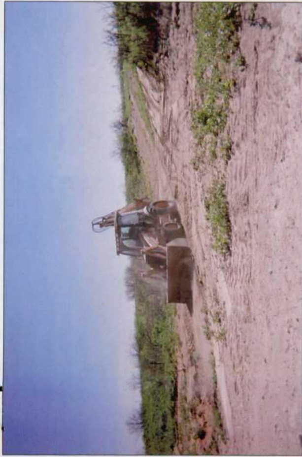
backfilling trench with imported soil
