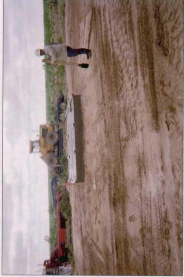
Backfilled site with new jct. box; clay ID plate in foreground
