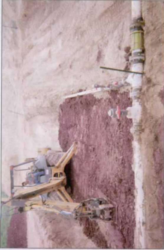
compacting clay
