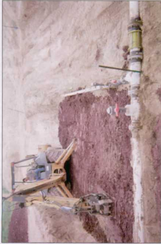
compacting clay
