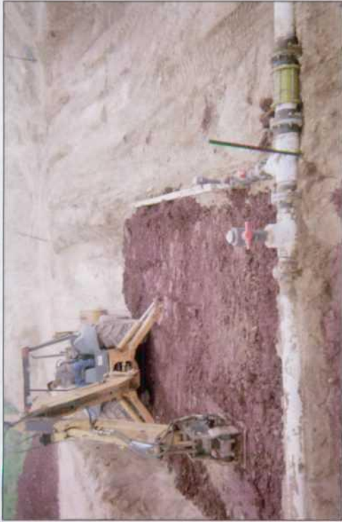
compacting clay barrier
