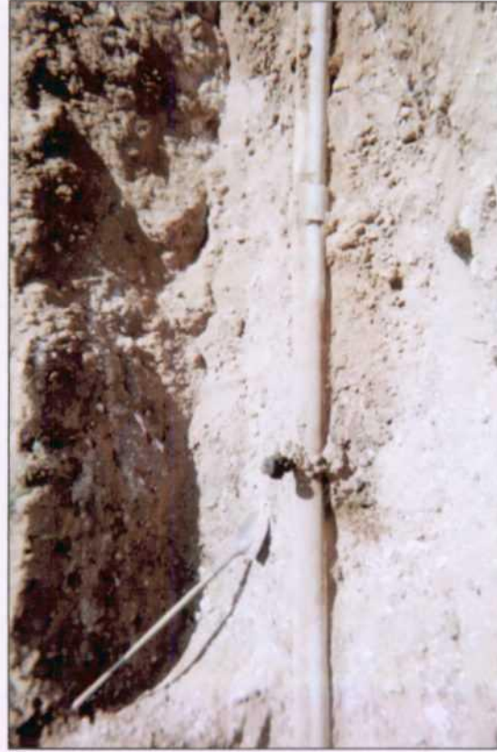
box removed, pipeline exposed with vent 8/30/2003
