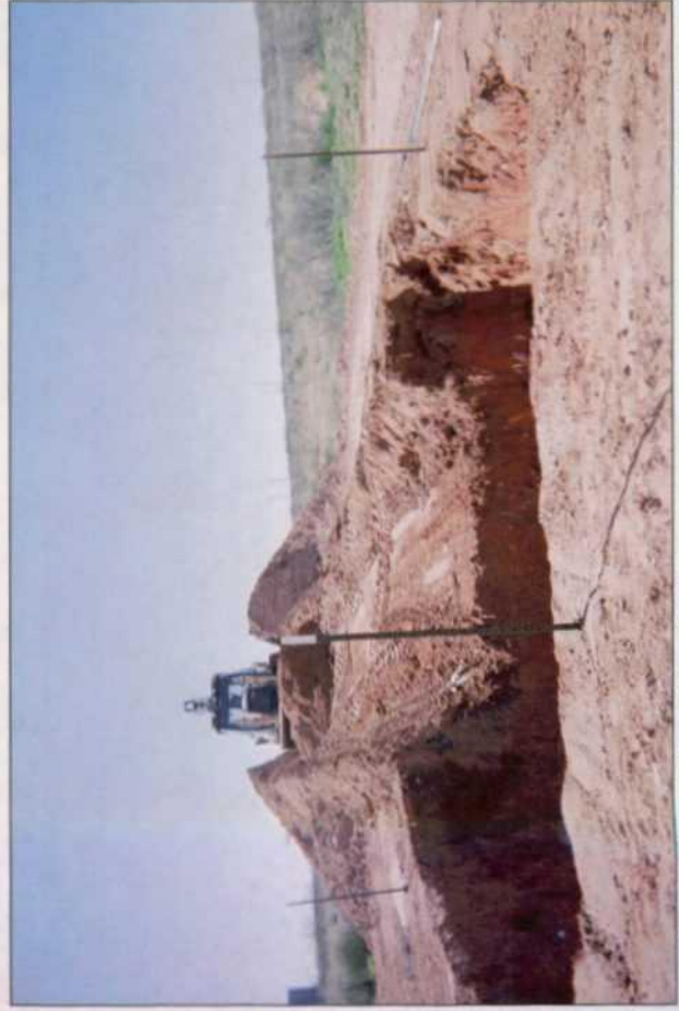
backfilling 20 x 20 x 12-ft excavation
