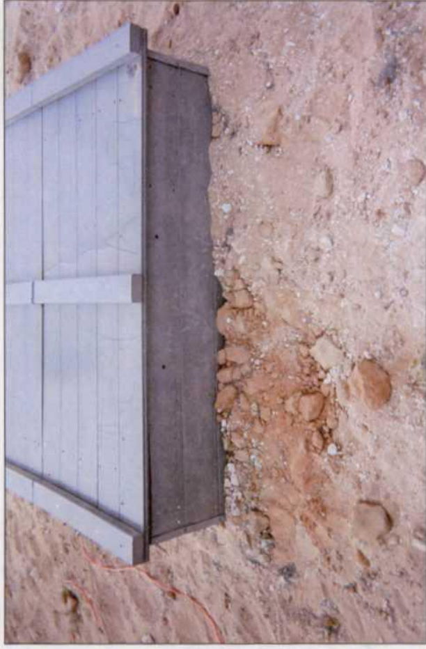
completed new junction box
