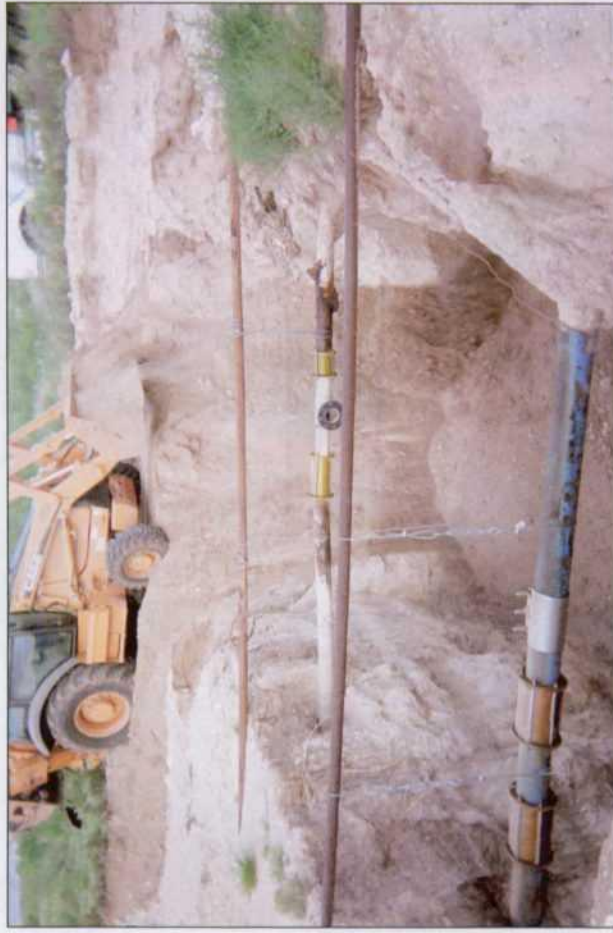
backfilling 10 x 12 x 12-ft-deep excavation
