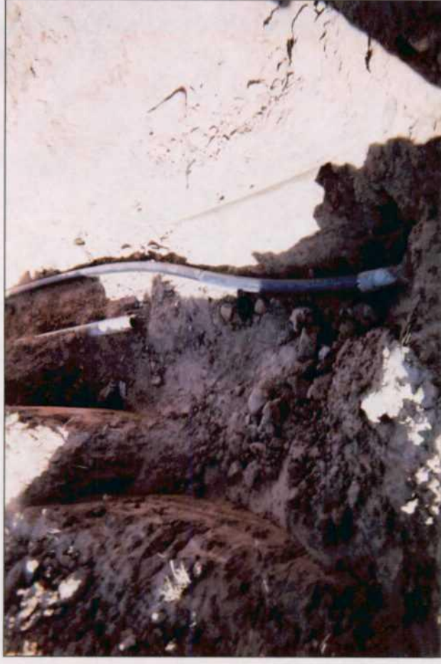
junction and box removed; pipeline replaced
