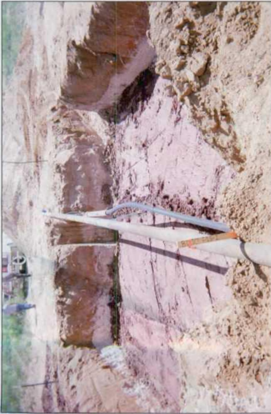
excavation with compacted clay at 6 ft BGS 5/28/2004
