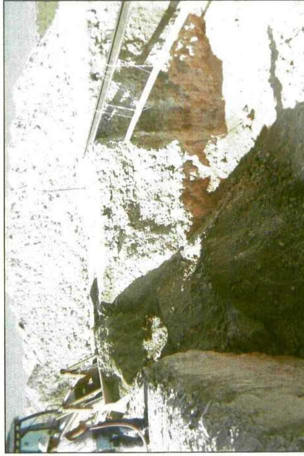
backfilling 30 x 25 x 12 ft deep excavation
