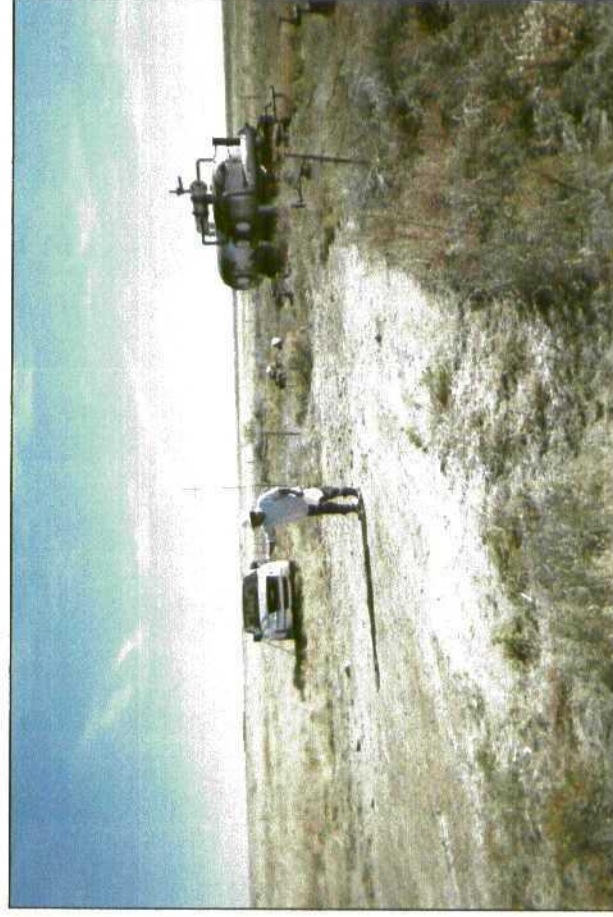
seeding disturbed surface after backfill
