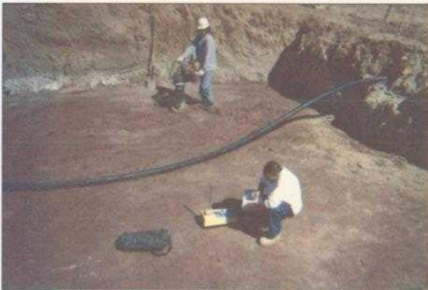
Compacting and Testing Clay Liner at 6 ft BGS 10/2/2003
