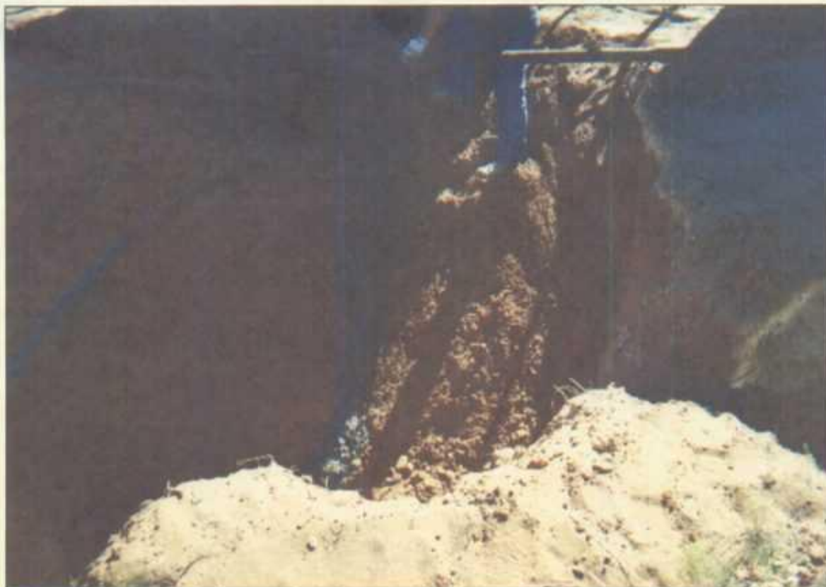
Repairing battery leak as crude and water spill into excavation
