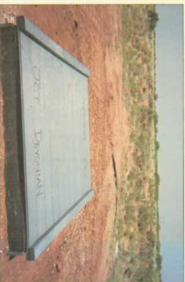
completed new watertight junction box 167 ft north
