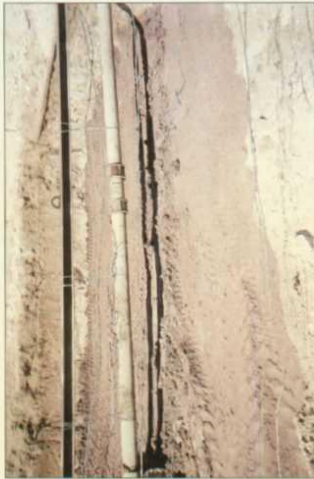
compacted clay at 6 ft BGS
