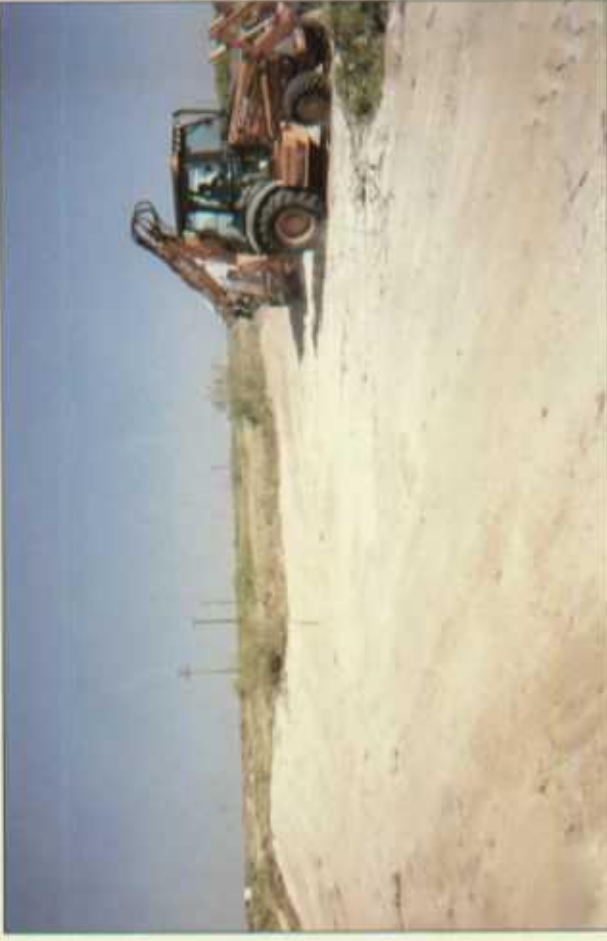
finishing backfill (looking east)
