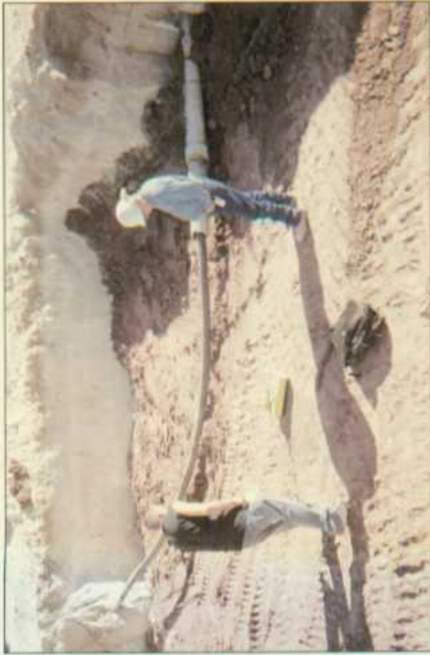
testing compacted clay
