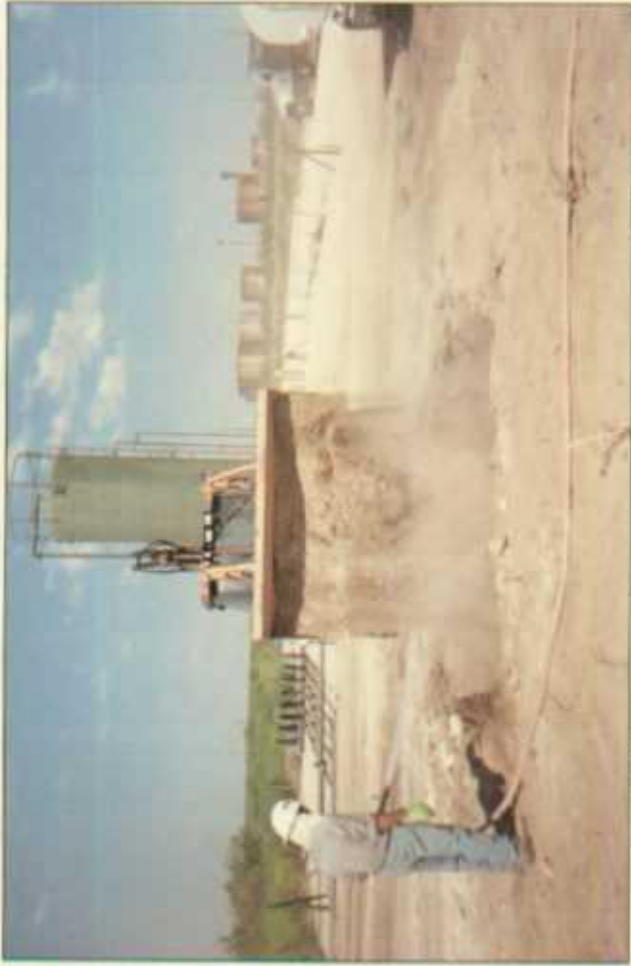
backfilling excavation
