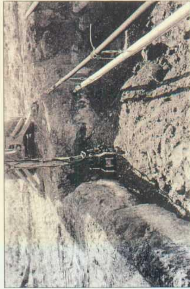
compacting backfill on top of clay
