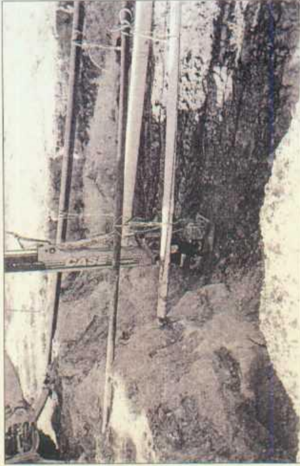
installing clay barrier at 6 ft BGS
