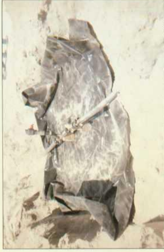
poly liner under new plumbing for new box 25 ft south of old box
