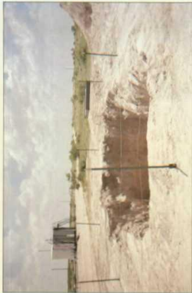
final 10 x 20 x 12-ft-deep excavation (looking south)
