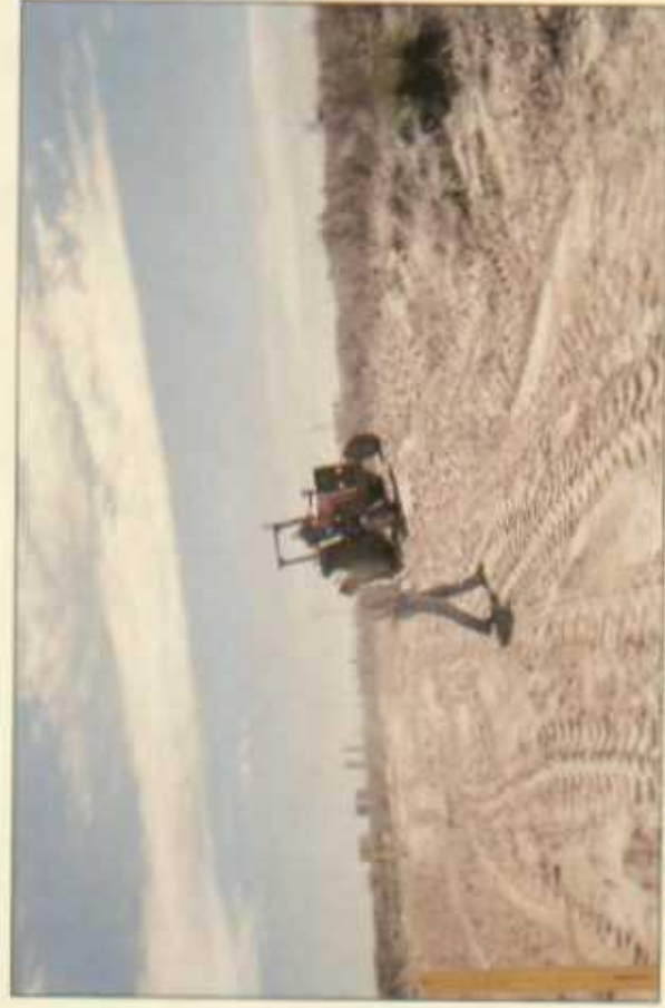
seeding disturbed surface at backfilled site
