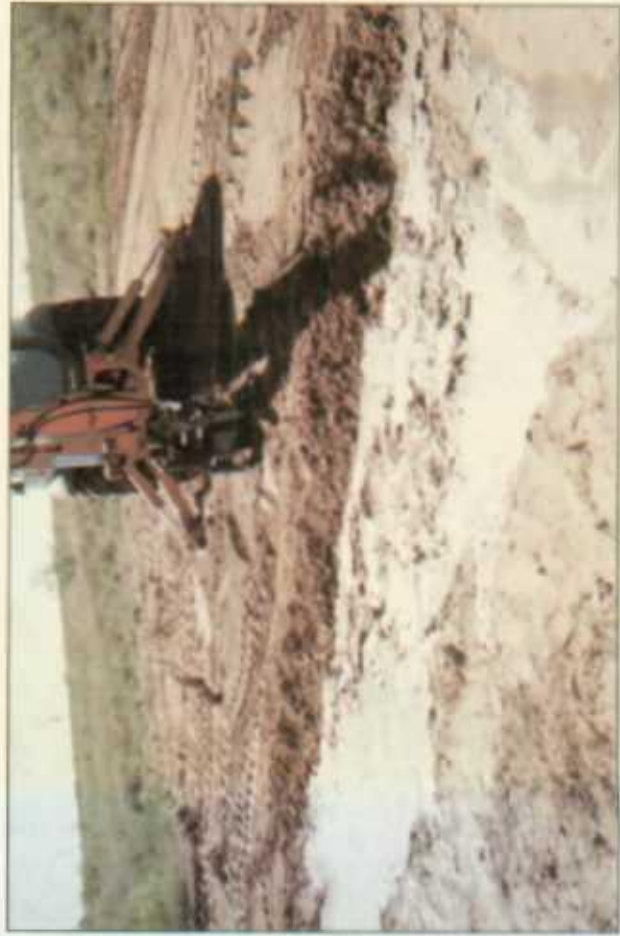
backfilling delineation trench
