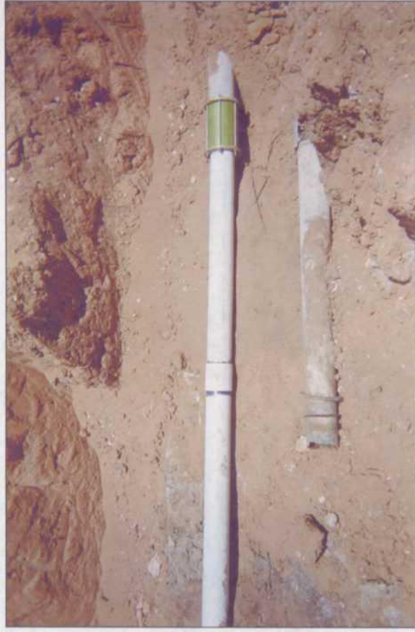
new plumbing; junction removed 7/16/2003
