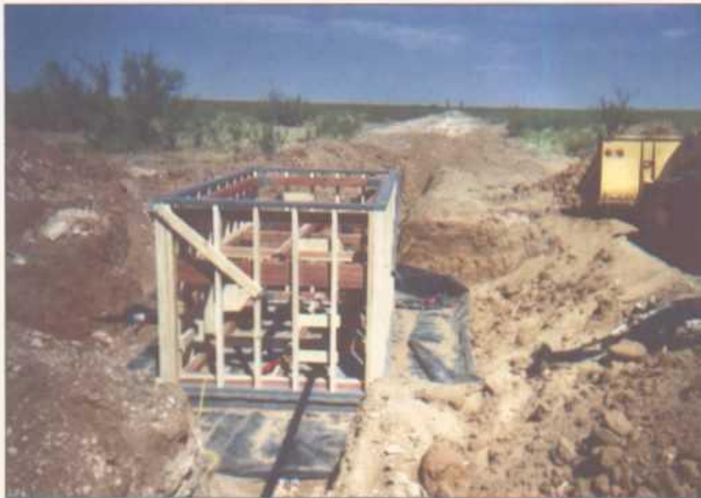
New Junction Box Construction 80 ft North
