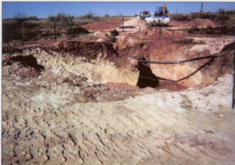
Excavation with Clay Liner
